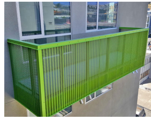
All of the railing was installed off of scaffolding.
