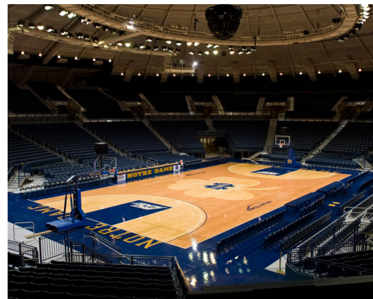
7,500 linear feet of architectural glass and aluminum railings were installed by our team.
