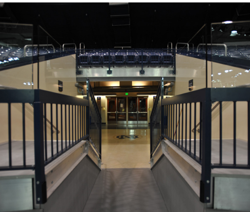
Stair units were included to allow fans to safely travel between floors.
