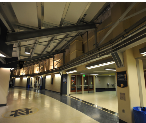
Structural raker beams provide usable walkways below the seating systems.
