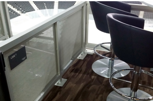
Private PCL loge level features custom aluminum railing with perforated panel infill
