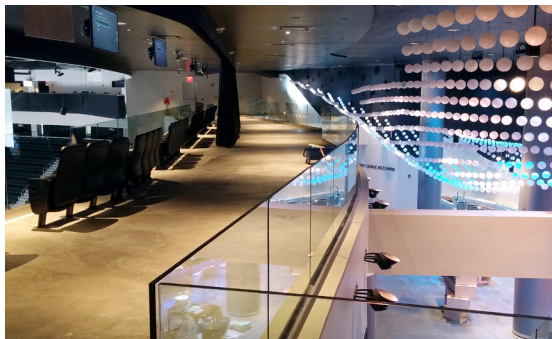
Track Rail with 3/4" laminated tempered glass was used on the Sky Lounge.
