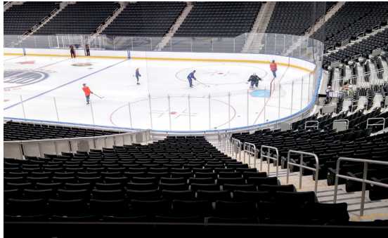
Aluminum Griprail with wifi boxes extending wifi capabilities throughout arena.
