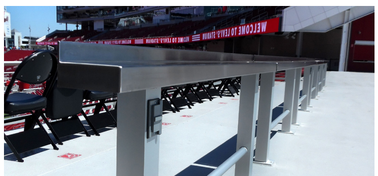
Tube posts with formed stainless steel drink surface & outlets
