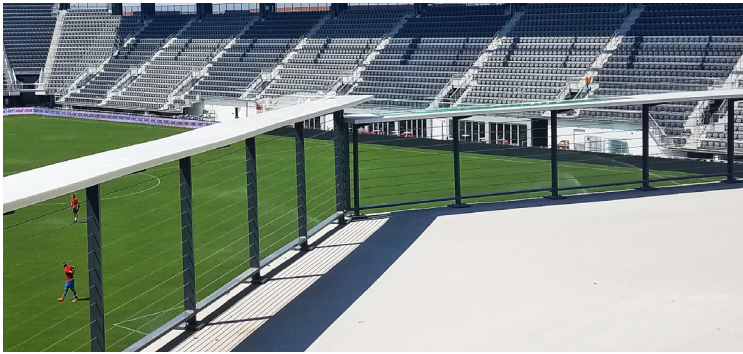
Custom Cable rail with solid surface top
