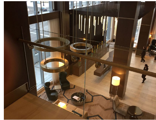
Point Series side mount with 36" high handrail.
