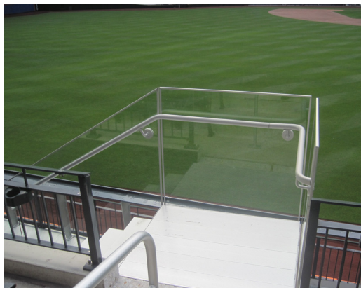
Track rail glass railing assures a clear view of the field.
