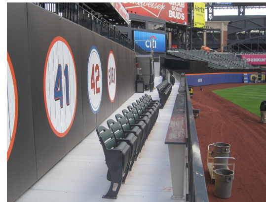
Ribbed aluminum flooring provides a rigid and safe walking surface.
