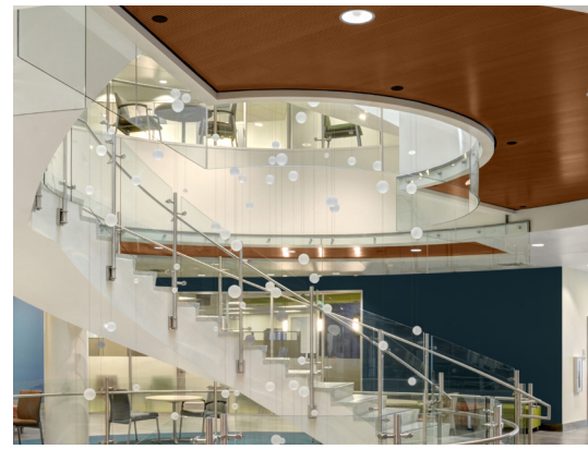
Point supported smoke baffle utilizes 3/8” glass illustrating form and function.
