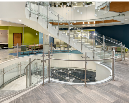
The top-mounted Equinox railing system has railing posts, along with steel post insert material, embedded into core-drilled holes in the concrete.
