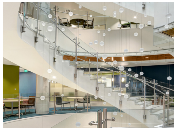
The circular staircase features a fasciamounted railing application, facilitated by attaching a 4x6” stainless steel mounting plate to a steel weld block.
