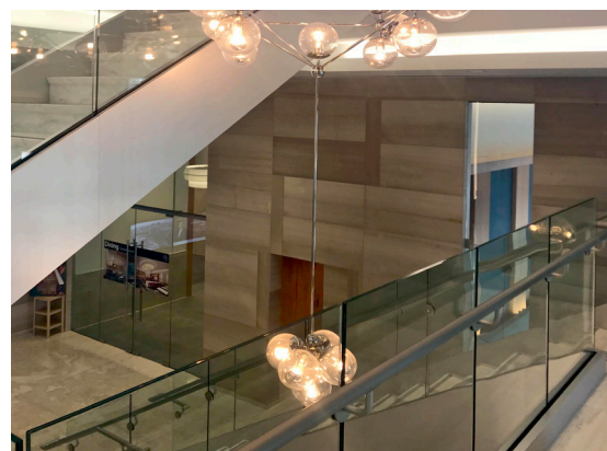
Clear, tempered, laminated glass with PVB interlayer and polished edges enhances the airy aesthetic.
