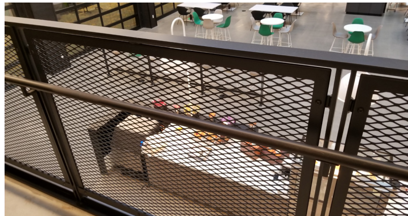
Metal infill panels with steel framing were custom designed by slitting & stretching metal sheets to create diamond-shaped infills.
