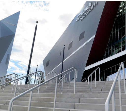
Anodized aluminum GripRail on exterior grand stairs entering U.S. Bank Stadium.
