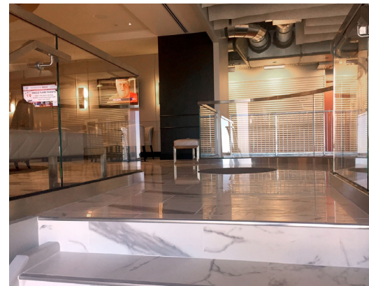
Clear, low-iron tempered glass with polished exposed edges and stainless steel top rail create a luxurious setting.
