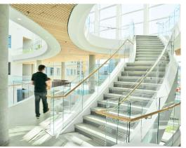
Custom-designed rolled and raked stainless steel cladding lines the building's three curved staircases, adding a perfect finishing touch to the space.
