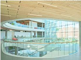
The building's stairs and curved overlooks feature 1/2" clear fully tempered monolithic glass, providing unobstructed views of the entire space.
