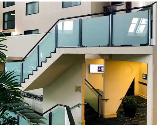
Custom glass railing found on stairs, overlooks and ramps utilized an opaque interlayer creating privacy within the pool area.
