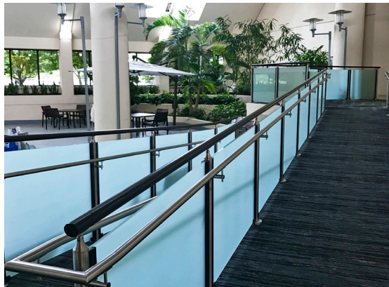
Top mounted glass railing features 1/2" clear laminated glass with opaque white PVB interlayer.
