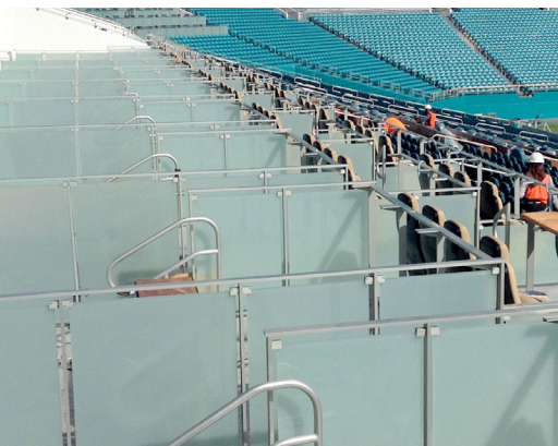
Custom post supported glass railing used in high-end 72 Club 'living room' luxury seating areas.
