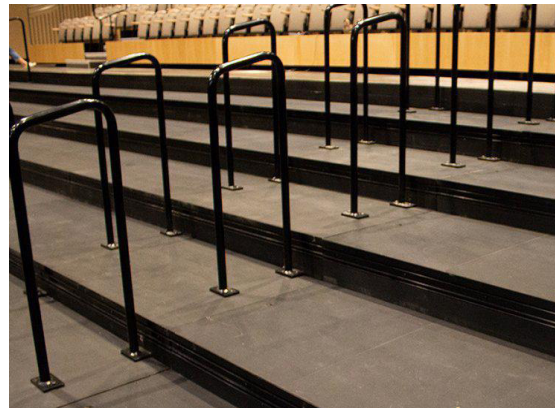
Six IBC Guardrails placed at each end of the Uplift extension offer enhanced safety and character.
