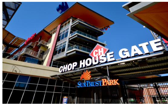
Track Rail utilized on multi-level balconies overlooking the Chop House Gate allowing for clear sightlines.
