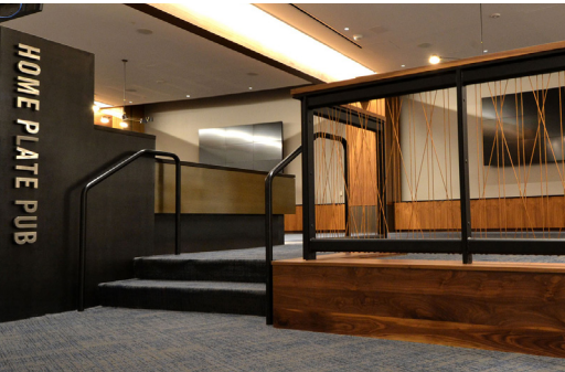
Home Plate Pub features a highly decorative cable railing with blackened steel frame.
