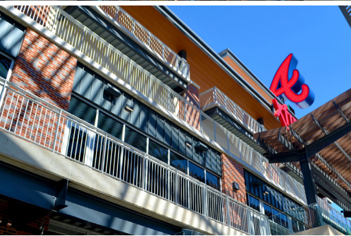
Anodized aluminum picket railing on balcony overlooks above the Terrapin Taproom.
