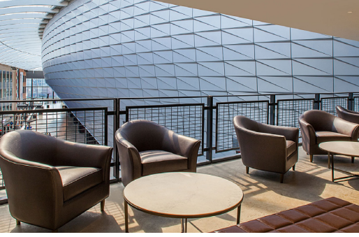
Black powder coated Gridguard railing with mesh infill lines this premium seating area.
