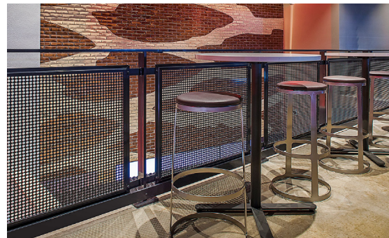
Black powder coated Gridguard™ railing with mesh infill found throughout the arena.
