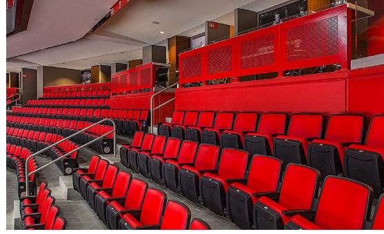
Custom Redwing Red Gridguard railing with perforated infill overlooking the arena floor.
