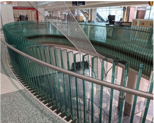
Sightline Commercial Solutions used 90 linear feet of high-end glass fin railing panels.
