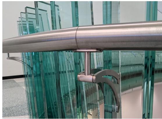
The glass fin railing panels are framed with stainless-steel handrail.
