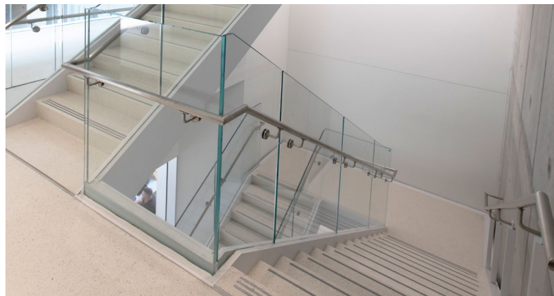
Tempered glass infill allows an abundance of natural light to flow throughout the space.
