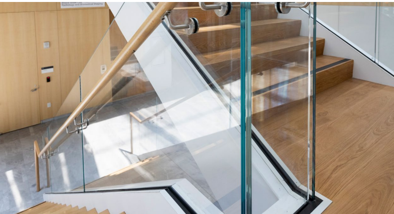
Glass nut Track Rail with post supported stainless steel handrail lines the staircases.
