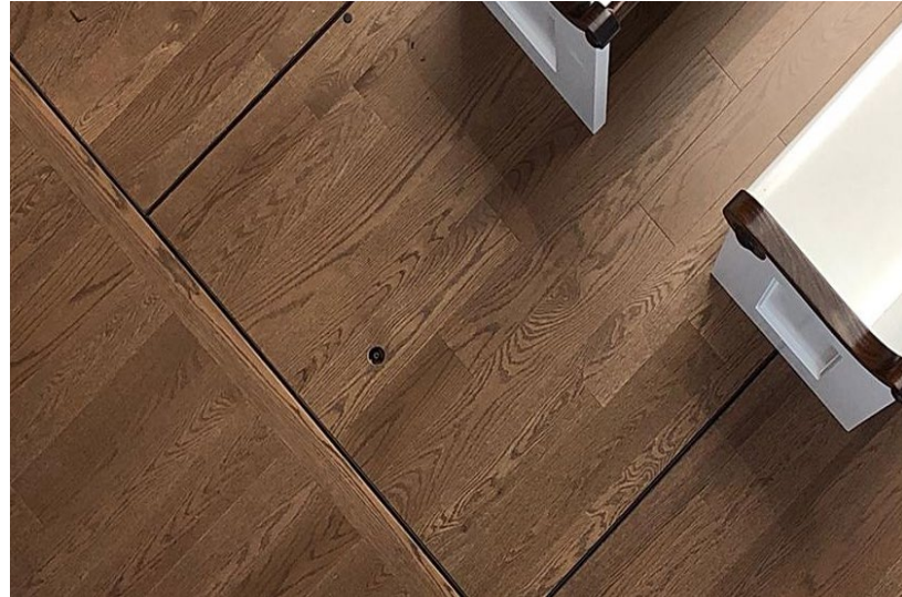
Custom built to fit perfectly into the existing space, the scissor-lift platforms allow the school numerous options for configuration layouts and expand the existing performance area to accommodate larger shows.
