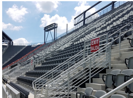
Horizontal Classic Picket Railing is face mounted into concrete in the vomitory areas and in front of ADA seating sections.
