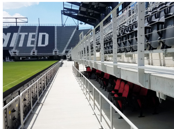
Tensiline Cable Railing can be found in front of the seating bowl, aisles, suites, overlooks & club patio. Courtesy Rail on the perimeter.
