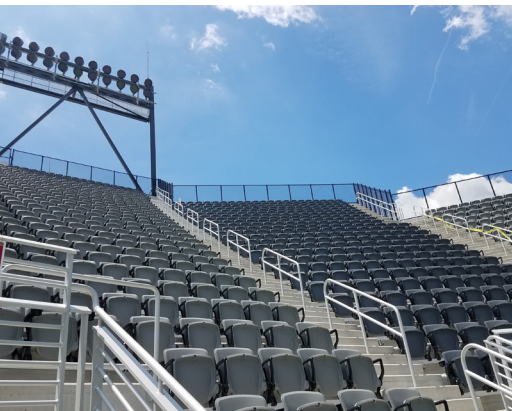
Griprail™ is floor mounted in the aisles, offering a graspable handrail for supporters as they walk.
