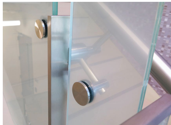
The laminated tempered glass has a .06” white opaque PVB interlayer between two 1/4” panels, creating an 80% transparent infill for a bright atmosphere.
