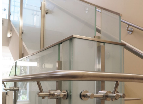
A u-channel top cap finishes the glass edge on the Line Series stair rail.
