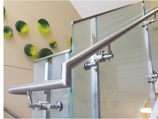
Stainless steel handrail is attached with a post mounted Line Series standoff.
