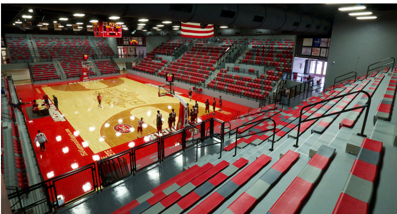
Sightline Commercial Solutions installed nearly 200 seating riser step units with handrail.
