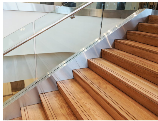
Custom fabricated sawtooth cladding conceals the base shoe and stringer along stairs and overlooks.
