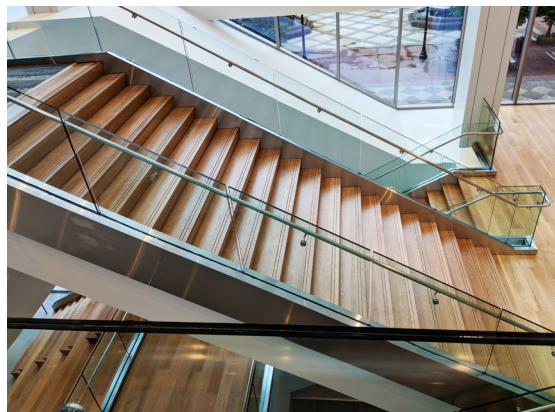
A wooden staircase guiding visitors to the second floor is lined with top mounted Track Rail glass railing.
