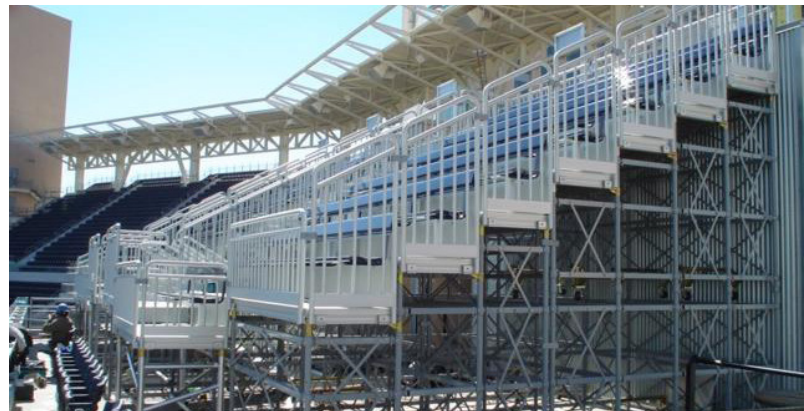
Changing the rise and run of the stadium, the riser section features larger tiers for a more spacious experience
