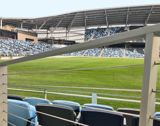
Tensiline railing with stainless steel cables is placed in front of fan seating areas, providing optimal views of the pitch.
