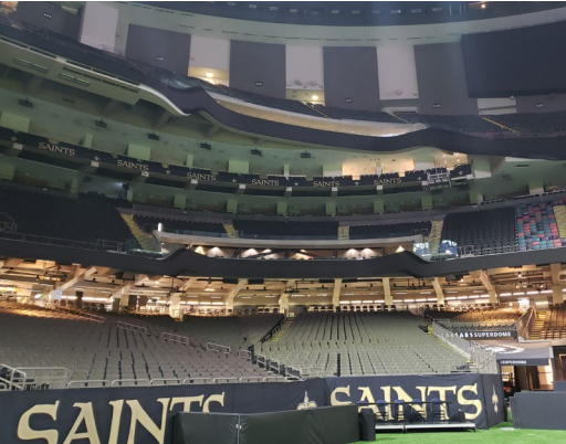
Glass railings on floating walls at the 200/250 Loge Levels and 500/600 Terrace Levels.
