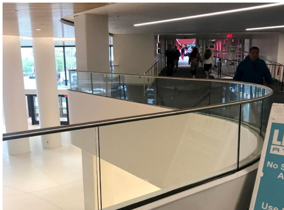
Specialty bent glass was also utilized for Track Rail on overlooks.
