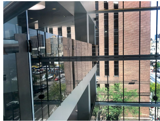
Fascia mounts for the Dot Series railing are almost completely hidden by the glass panels.
