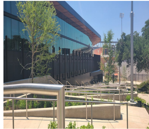
Handrails used around the arena.
