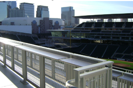
Gridguard mesh railing with drinkrail attachment found throughout ballpark.
