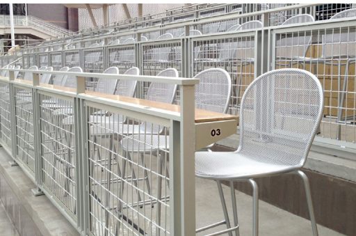
Custom Intercrimped wire mesh railing within U-Edge border.
