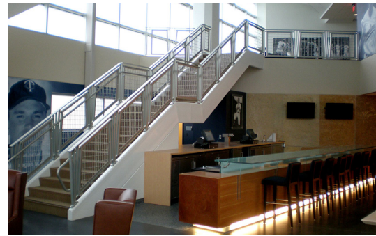
Gridguard aluminum mesh railing within interior suite areas.
