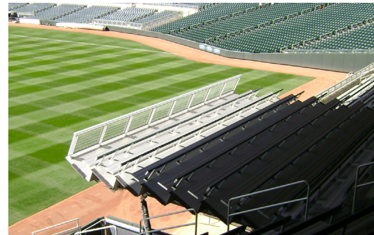
Operable seating platform acts as lift gate allowing vehicles onto the field.
