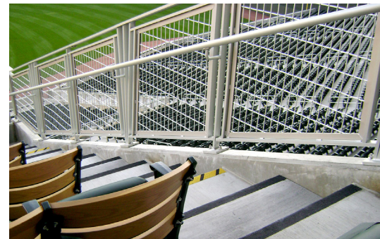
Gridguard railing system with intercrimped mesh infill and custom post configurations.
