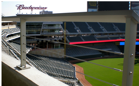
Tensiline railing with stainless steel cable infill at front of fan seating areas.
