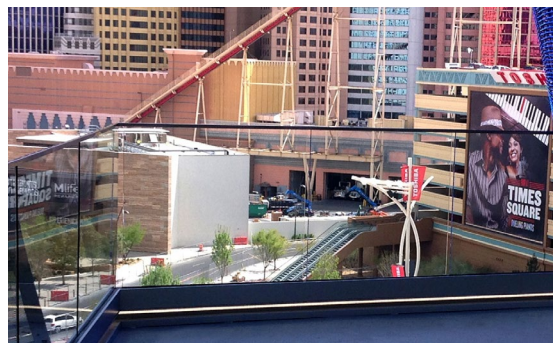
Custom-engineered base shoe glass railing system with LED lighting.
