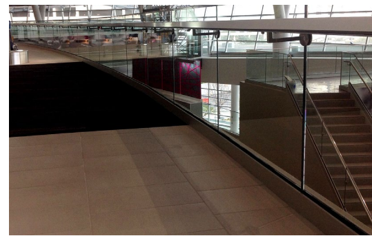
Custom drink rails with stainless steel supports friction-fit to 1/2" tempered glass.
