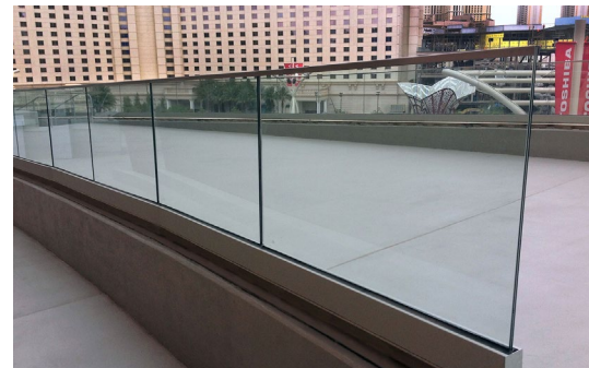
Front side of the custom LED lit C-channel base shoe glass railing system.
