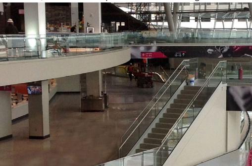
Glass base shoe railing on stairs and balcony overlooks throughout concourse levels.
