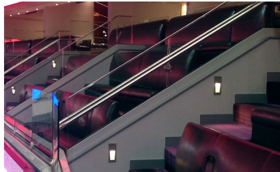
Glass base shoe railing with stainless steel handrail dividing suite areas.
