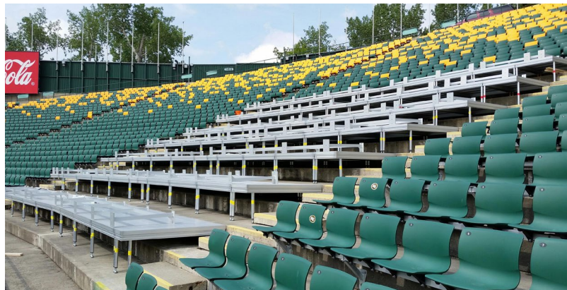
Stadium seats in two main sections were permanently removed for the 2016 season and replaced with a customized version of Sightline Commercial Solutions' all-aluminum SC97 platform system.
