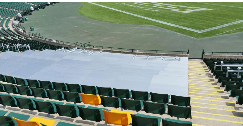
By implementing these specialized viewing decks, the physical "assigned" space for a single spectator was increased from around 4.5 square feet to an average of 8 square feet.
