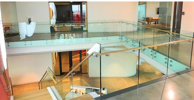
On the overlooks, Point nodes are mechanically fastened to a steel angle support with weld studs, allowing for openness.
