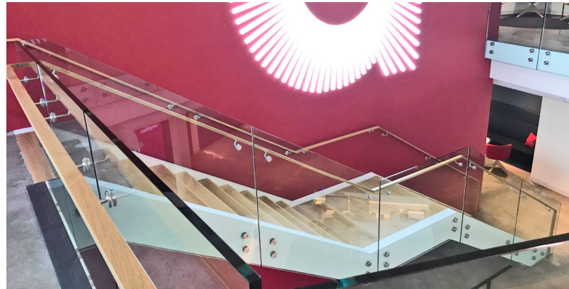
Wall and glass mount handrail lend sleek support for staff and visitors throughout the office.
