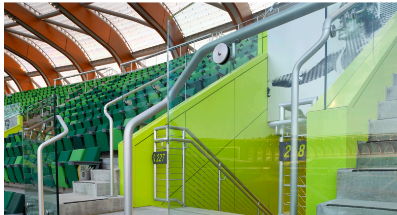
Anodized aluminum guardrail with post-supported clear glass panels delivers optimal sightlines for spectators.
