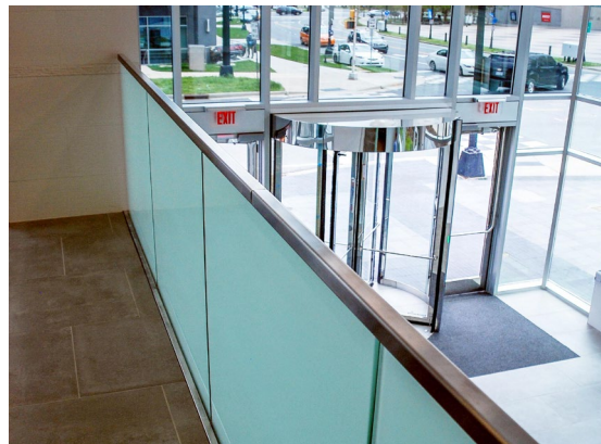
Track Rail with 1/2" frosted laminated glass adds stability, and a stainless steel U-Channel top rail enhances the building's modern aesthetic.
