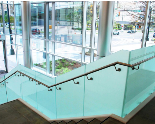
Track Rail and Point Series are featured as complementary railing systems that enhance the lightness of the space.
