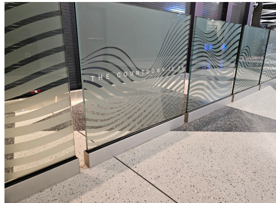
Point™ supported glass railing and custom-patterned etched glass ensured a sleek and modern aesthetic.
