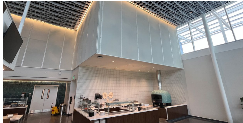
Perforated aluminum sheet panels are installed over the kitchen/dining areas.
