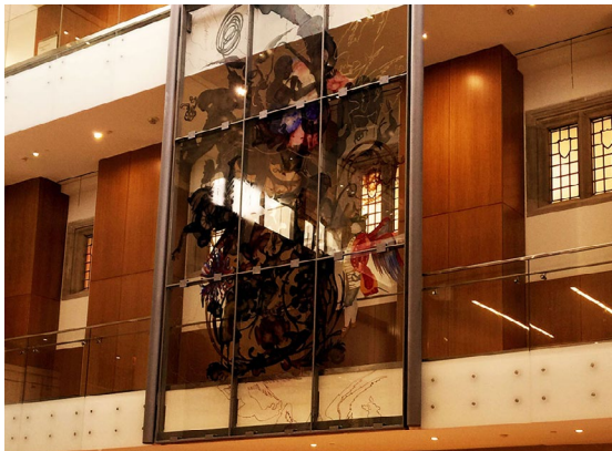
The Point series systems was chosen for the renovated 3-story atrium, eliminating the need for vertical balusters.
