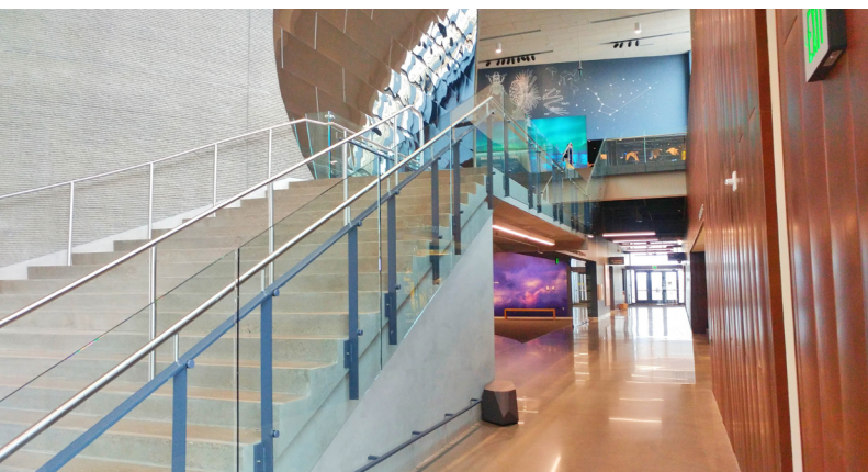
Fascia mounted posts attached to concrete using Hilti Hit-z epoxy anchors accommodate the drop side glass overhang.
