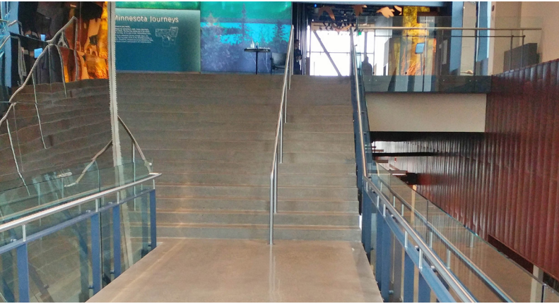
Post Rail with 1/2" tempered clear glass infill ascends the monumental staircase leading to the second-floor exhibit hall.
