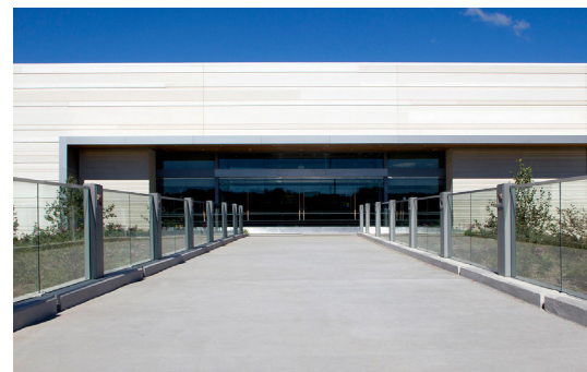
1/2" clear laminated tempered glass with a 060 SGP Interlayer.
