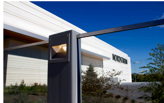
Pedestrian Bridge - Base Shoe glass railing with custom painted lit bollards.
