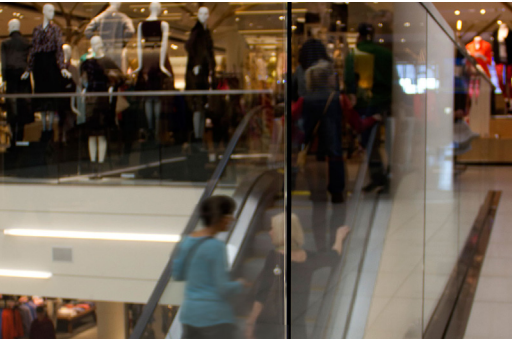
Aluminum Base Shoe interior glass railing.
