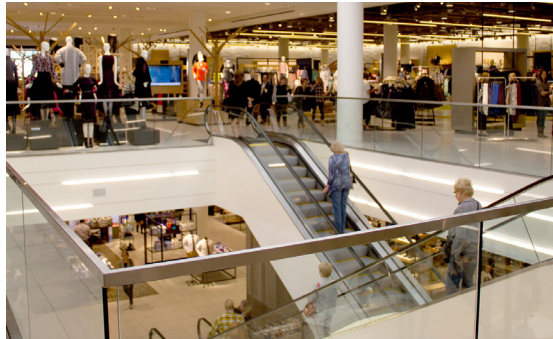
Interior Base Shoe glass railing on balcony overlook with 304 stainless steel top cap.
