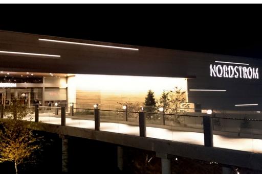
Pedestrian Bridge - Base Shoe glass railing with custom painted lit bollards.
