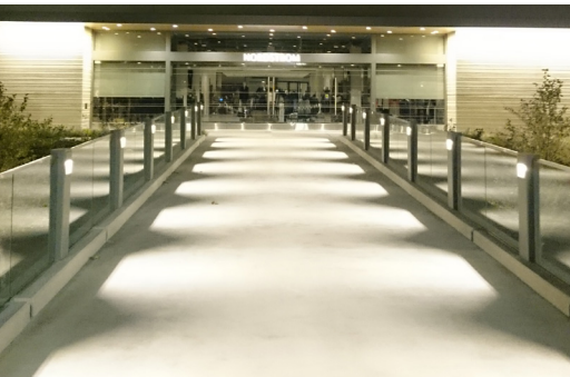
Exterior Base Shoe glass railing with custom painted lit bollards.
