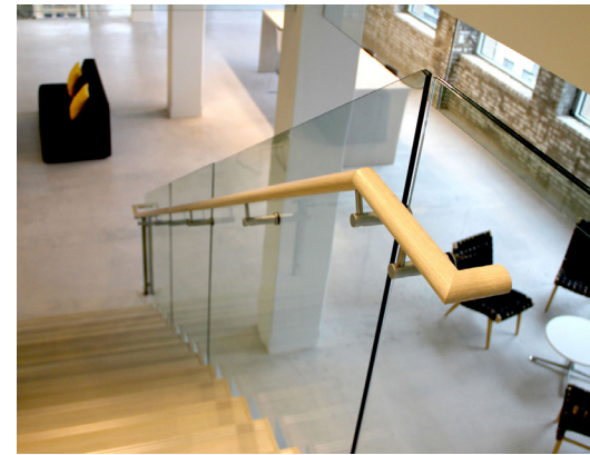
Custom bleached white oak wood handrail.
