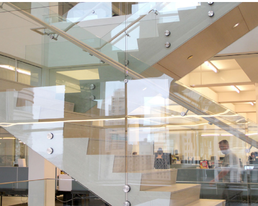
Point series utilized on multilevel staircases.
