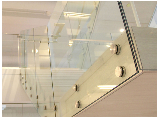
1/2" laminated tempered glass with a 060 SGP Interlayer.
