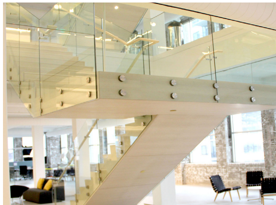
Eliminating the need for vertical balusters allows for openness and clean sight lines.
