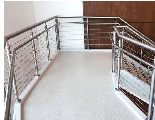
Post-mounted handrails are continuous from the staircase to landings, providing a seamless look.
