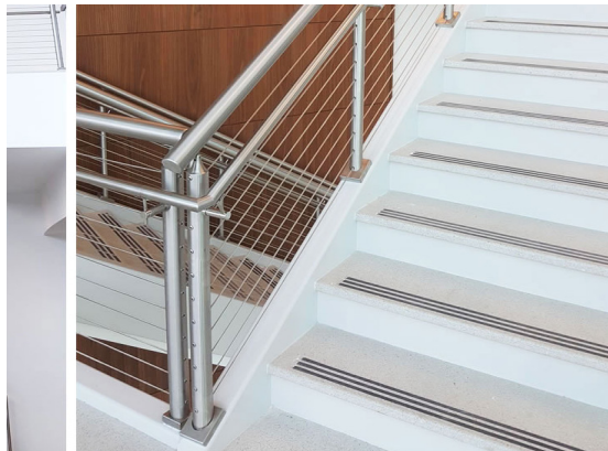
For added safety and security, double posts were installed at all breaks and corners.
