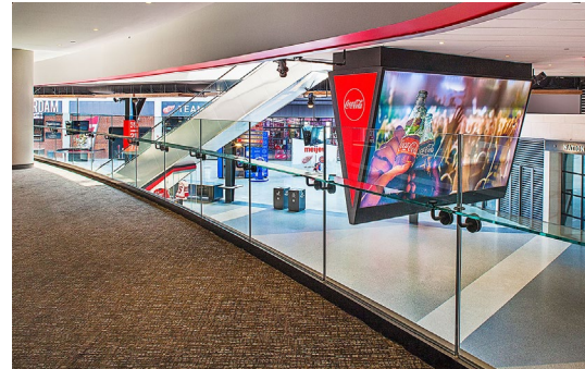
Top mounted Gridguard railing with custom drink rail utilized on the suite level bridge.
