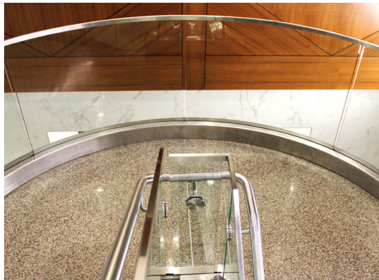
This curved landing required rolled aluminum base shoe, cladding, top cap and glass to achieve the desired tight radius.
