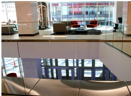
The newly renovated seating area above the updated main lobby utilized Track Rail with formed top cap & 1/2" clear tempered glass.
