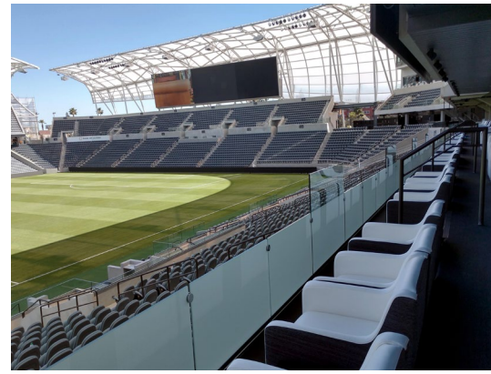
Split panels of Mist Fog Glass set within the Track Rail™ system allow for transparency from both sides to optimize views from The Directors Box.
