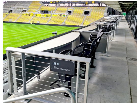
Loge Boxes feature crescent-shaped drink rails with phenolic modesty panel infill allowing fans to enjoy beverages without missing the action.
