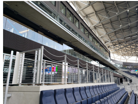
Clear tempered, laminated glass with SGP interlayer offers unobstructed views and a luxurious touch to the stadium.
