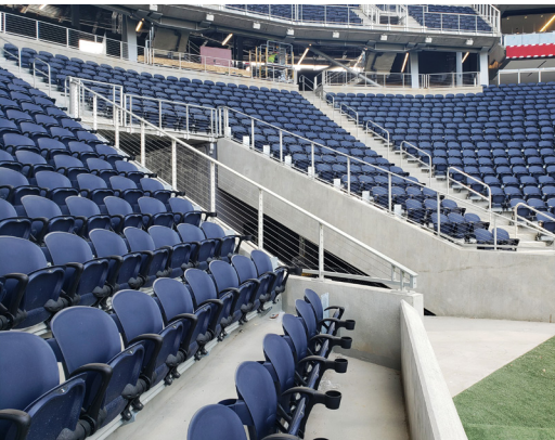
Griprail™ and Tensiline™ railing are featured throughout the seating bowl to ensure safe movement for fans.
