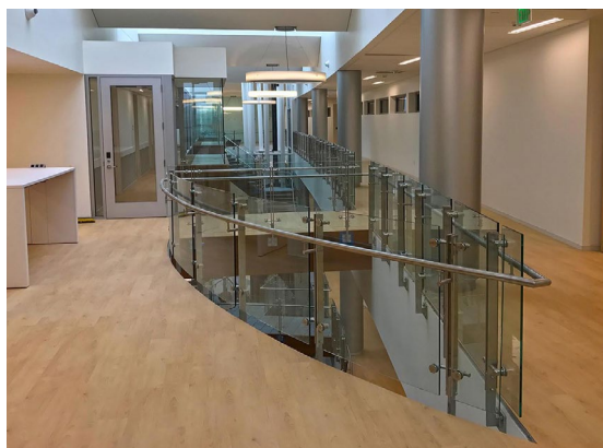
Overlooks feature a radius application with post-mounted stainless handrail.
