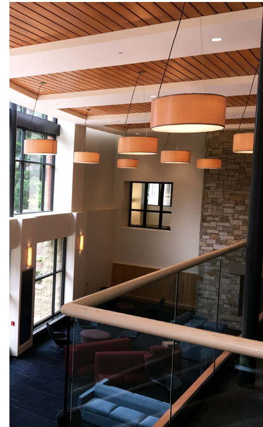
Trim was curved to the same radius as the railing. Custom jigs were created to fabricate the coping in-house.
