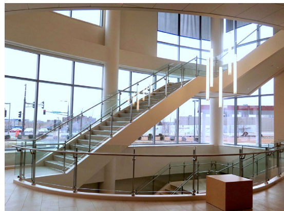
1/2" clear tempered glass allows light to flow through multiple levels of the facility.
